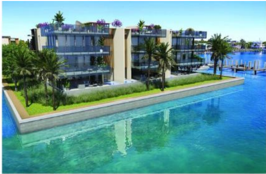
Groundbreaking of Forté Luxe, Luxury Waterfront Community Groundbreaking of Forté Luxe, Luxury Waterfront Community (Forté Development)
