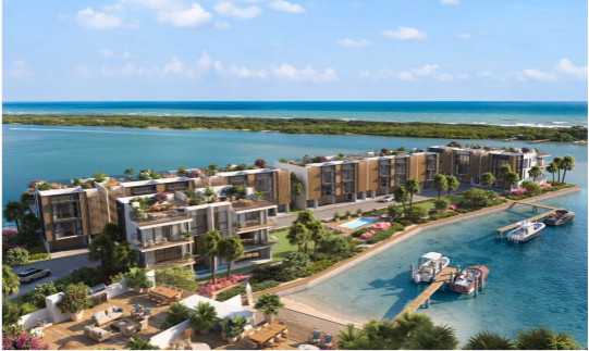
The multi-level residences are located on a peninsula that juts into the Intracoastal Waterway. Courtesy of wearevisuals.
